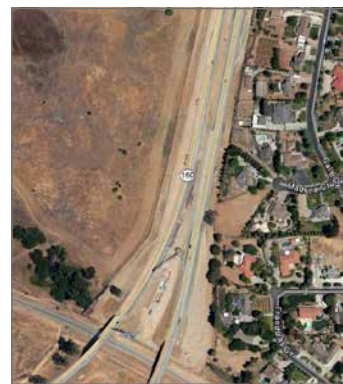
Bridge and road construction
